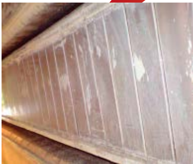
BEFORE installation of Victory IR system
